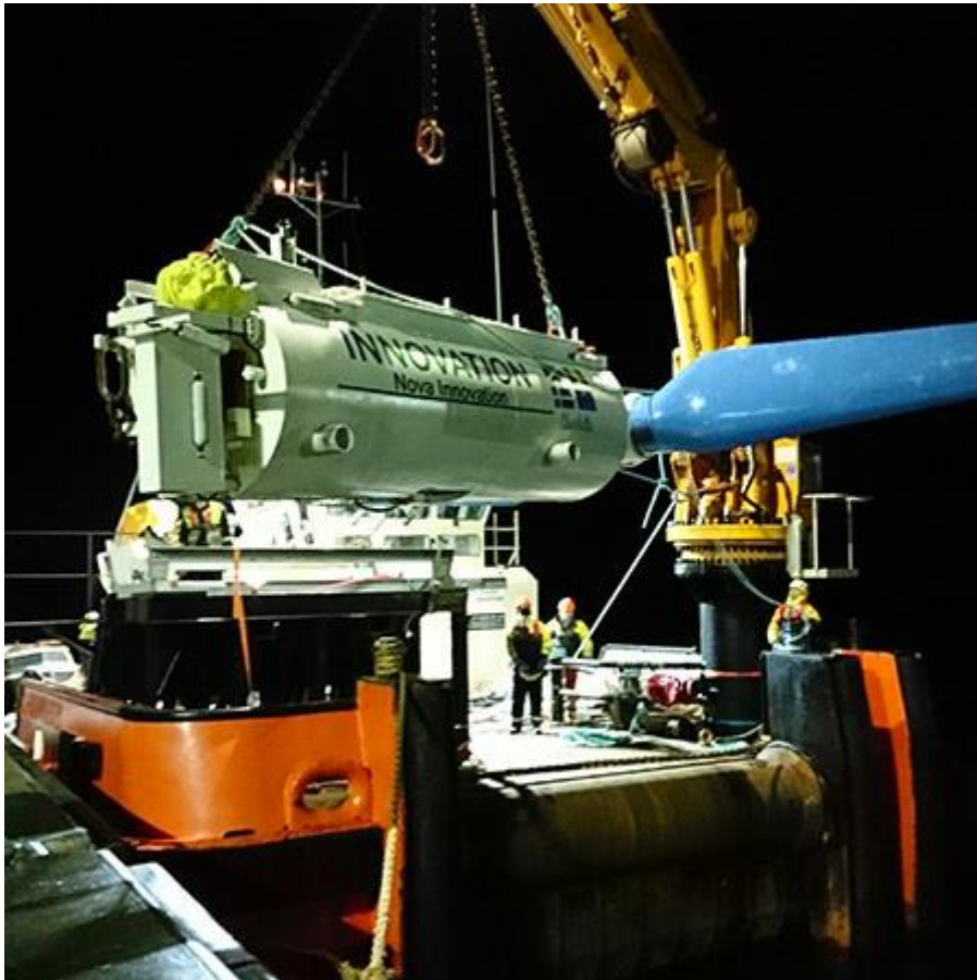
FIGURE 6.4 DEPLOYMENT OF A NOVA M 100 -D TIDAL TURBINE FROM MULTI-CAT VESSEL
